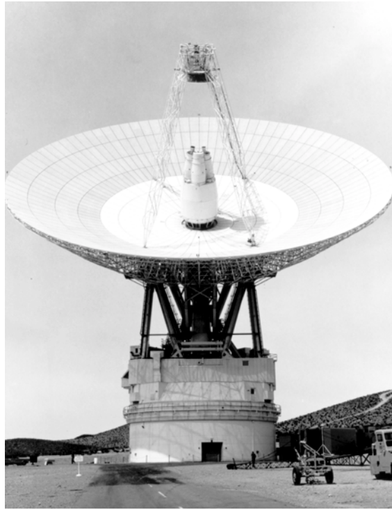
Fig. 5-9. Tricone installed on the 64-m antenna.
